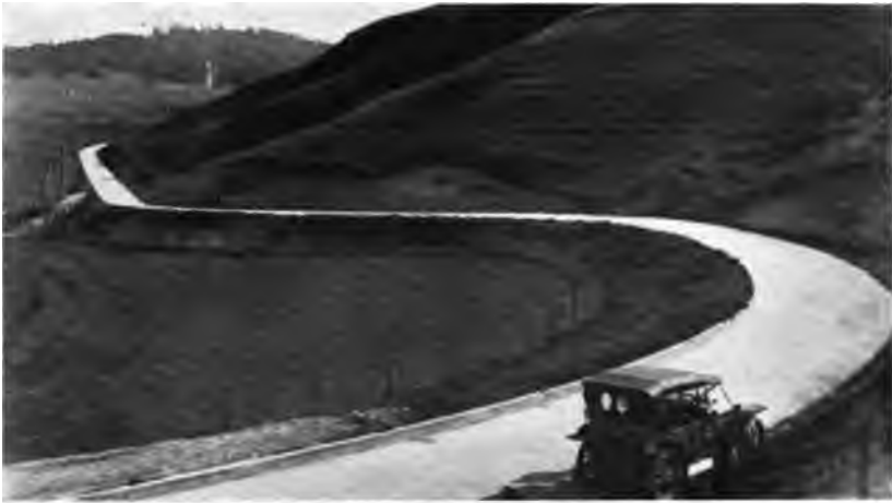
On the Santa Cruz lateral of the State Highway, showing concrete curbing.
